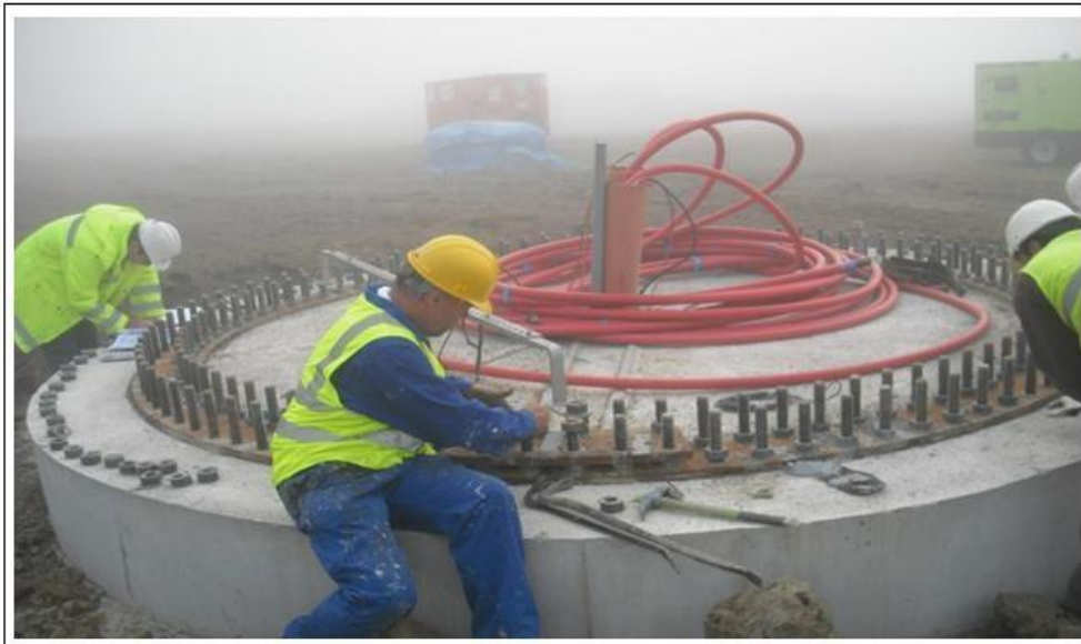
Figure no. 71: Derived foundation construction
