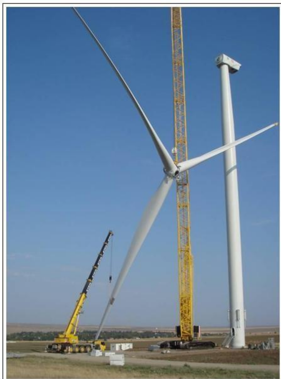
Figure no. 75: Installation of the assembled hub and blade on the wind turbine pole
