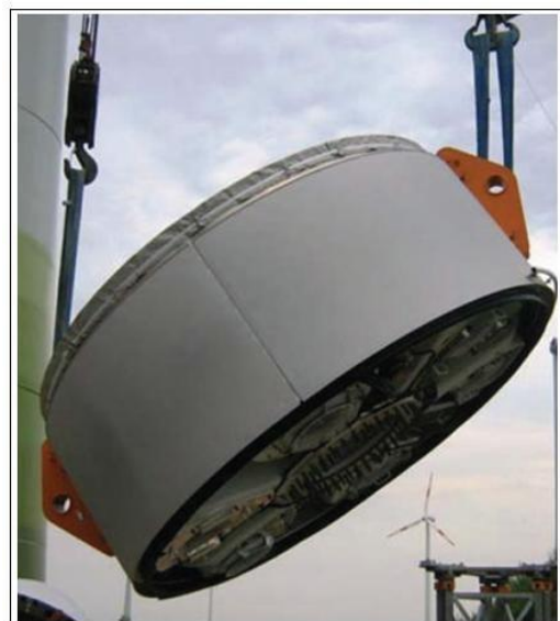
Figure no. 73: Installation of the gondola
