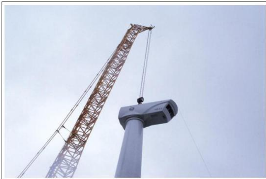
Figure no. 74: Lifting the wind turbine
