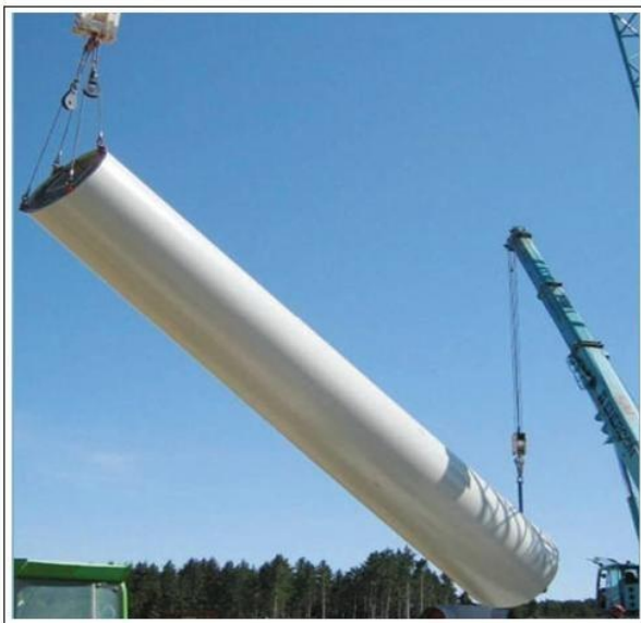
Figure no. 72: Lifting a column segment
